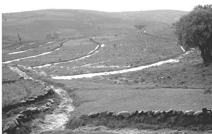
Fig.5 Graded bunds / banks (S3), graded ditches and waterways (S4) to drain excess water. Ethiopia. (Photo H. Hurni)
