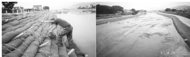
Coir logs - lake bank stabilisation in Switzerland
