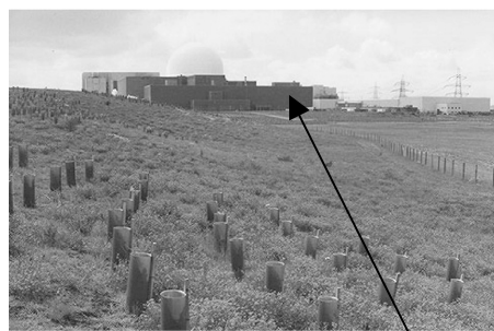
Fig. 2 12 months after application (note untreated brown area indicated in front of the power station)
