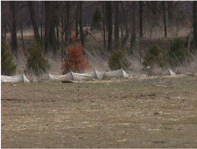
Plate 18. Silt fence
